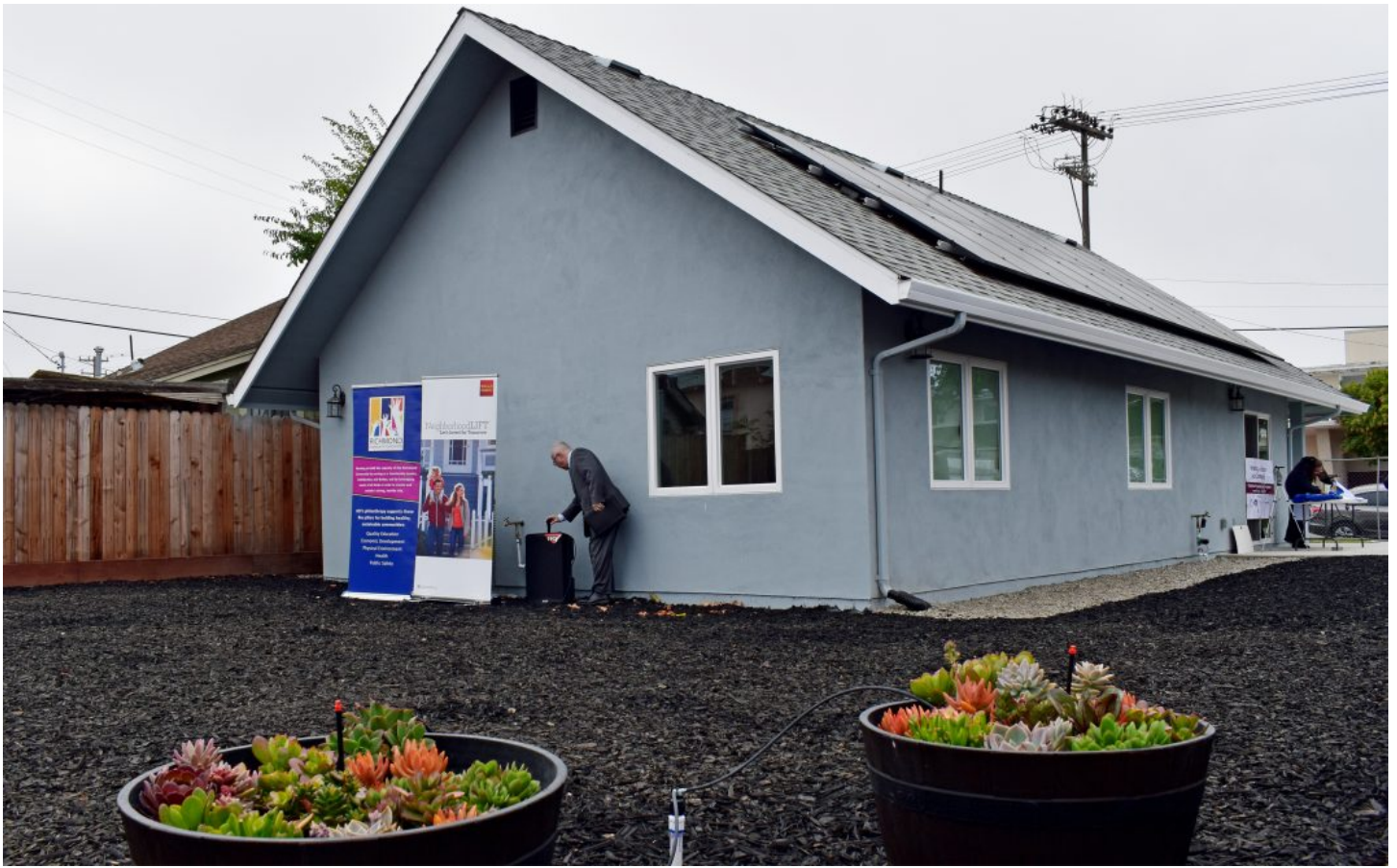
Back yard of the newly built house at 1025 Florida Ave.
